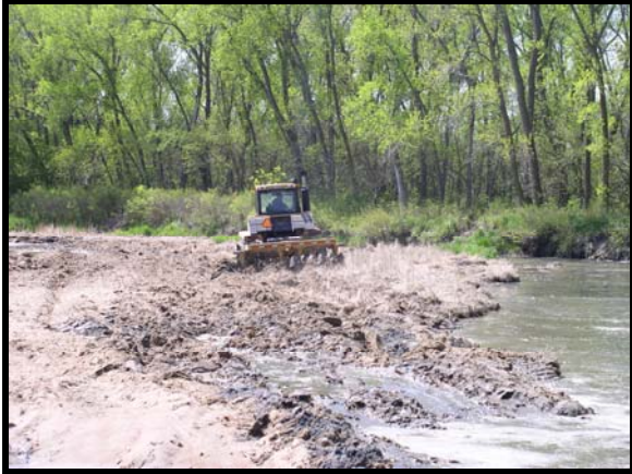
Deep disking of high sandbars on the Republican River has increased the scouring effect during high stream flows.
